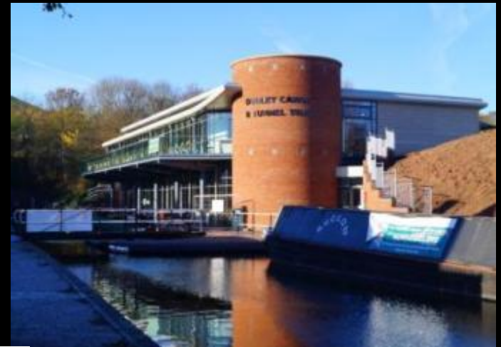
The New Portal building 2016
