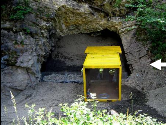
Loose Rock Infill to daylight gallery
