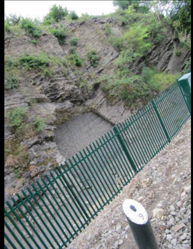
Loose Rock Infill to daylight gallery
