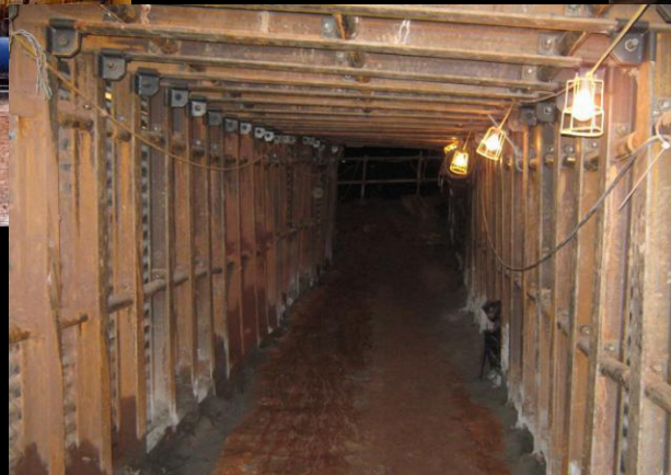
Heavily Shielded inspection Tunnel
