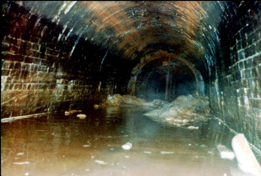
Castle Mill end of tunnel
