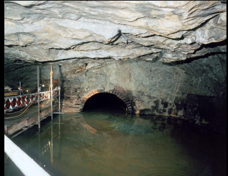
Step Shaft Mines end of tunnel
